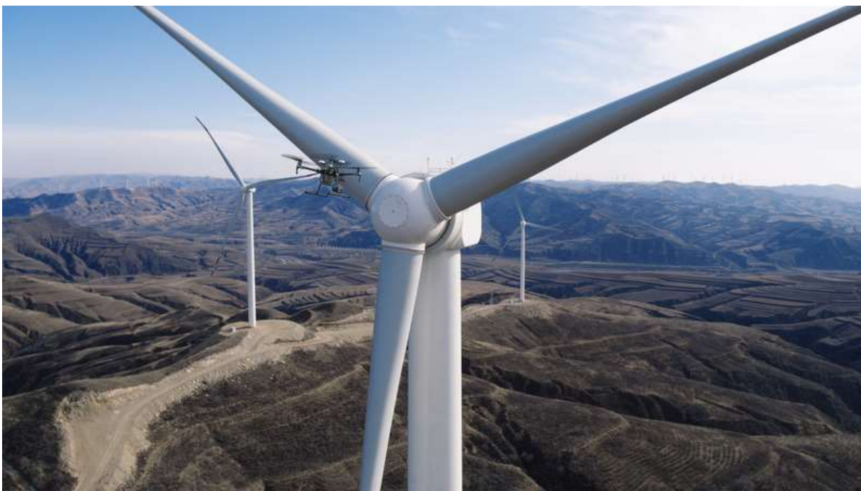
With the ability to watch inspections remotely, engineering teams are able easily manage global energy assets
